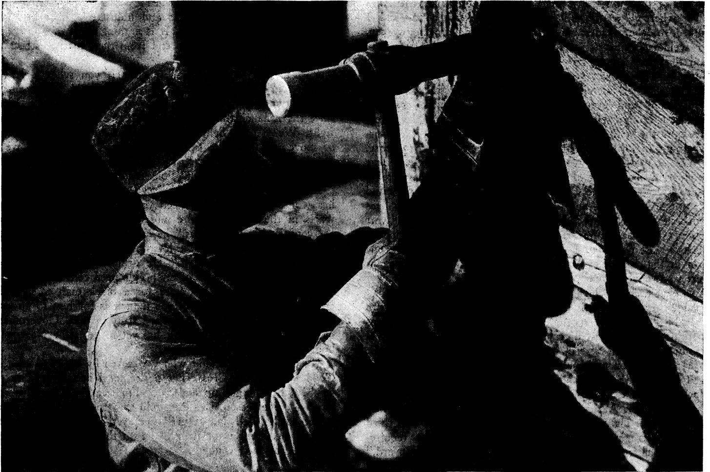
A Negro worker calking the seams of a reconditioned barge
