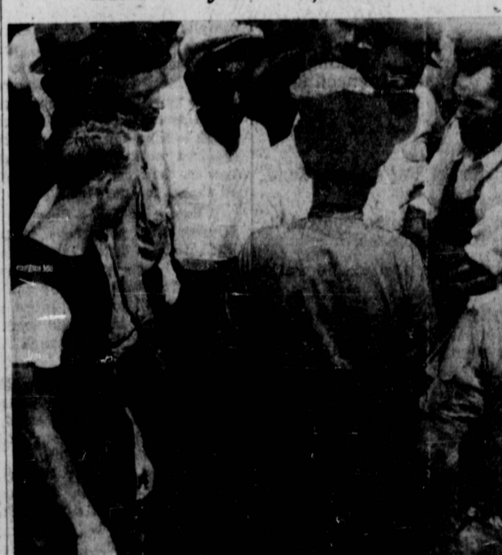
A group of WPA strikers at the Deephaven Bridge Project laying down the law to a cop. When the argument ended, the project remained shut tight!
