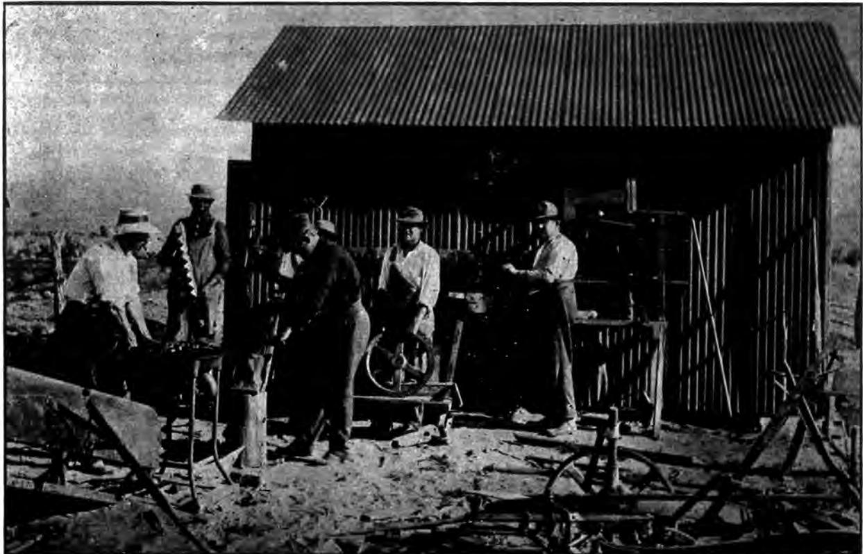
The first machine shop established at Rancho Llano del Rio was a small affair, where most of the work was done out of doors. Here repairs were made of agricultural implements and transportation machinery. The versatility of the colonists is a source of continual surprise.
