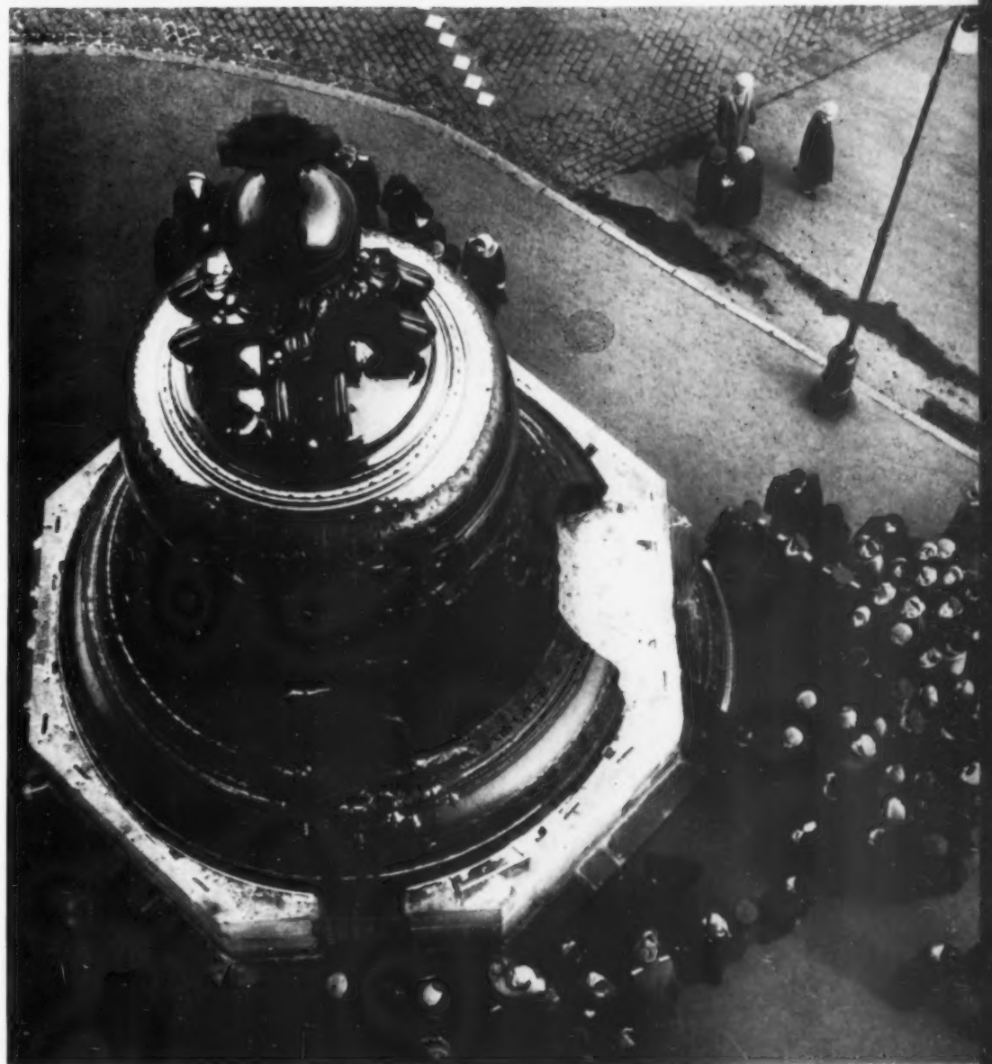
The Kremlin has two outstanding monuments of old Russian casting art. The King Cannon above weighs 40 tons and was cast in 1586. The King Bell at the right weighs 200 tons and was cast in 1735. Shortly after its completion a large section of the bell was broken off during a fire.
