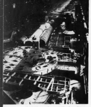
Overhead view of an assembly of a walking excavator at Dniepropetrovsk metal-working plant.
