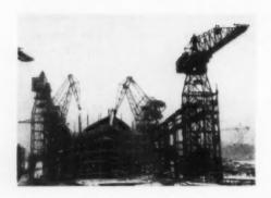
This huge skeleton framework rearing up above the scaffolding in a Leningrad shipyard is the hull of the first atomic icebreaker. The eighty-ton steel sections are lifted by tower cranes, placed gently in position on the stocks, ready for welding, to form part of the assembly for the stern and upper deck.
