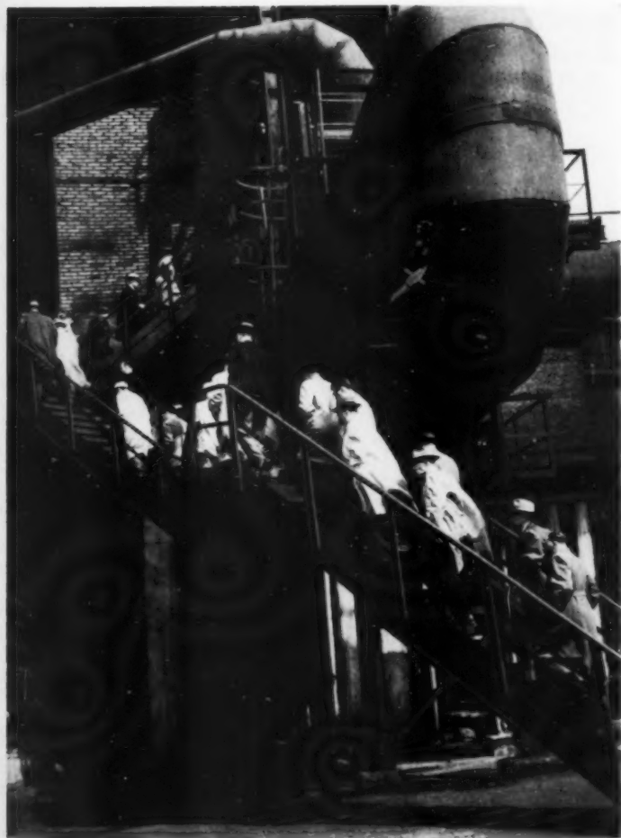
THE VISITORS FROM THE USA FIRST INSPECTED THE RECORD-SETTING BLAST FURNACE.
