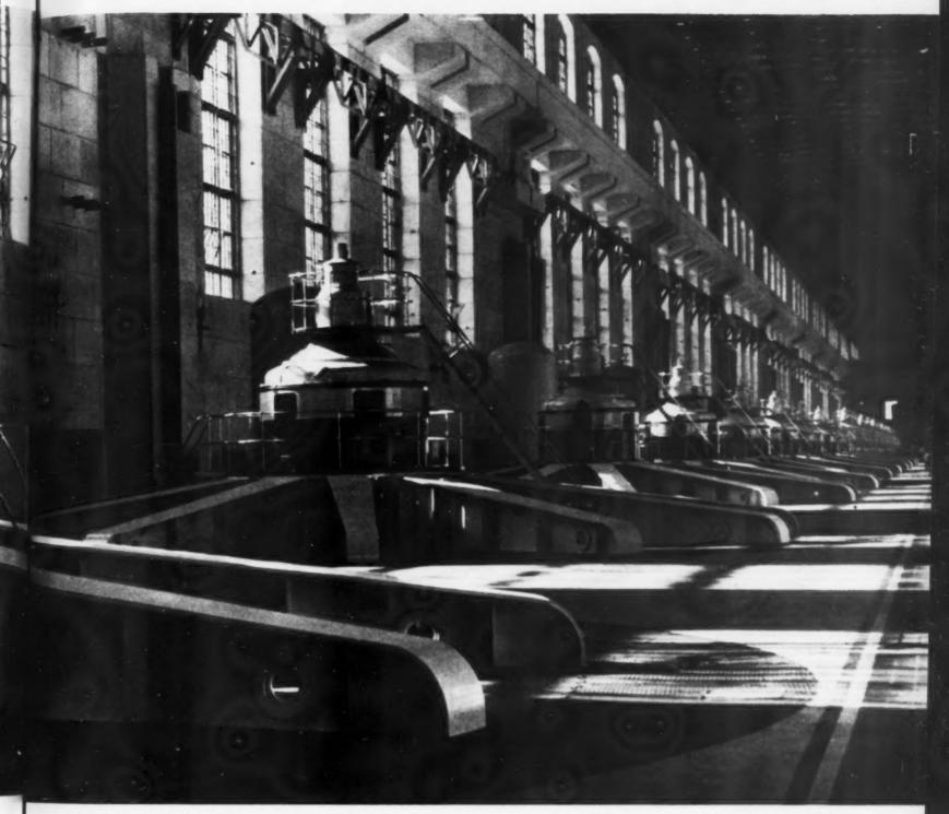
TWENTY TURBO-GENERATORS OPERATE IN THE POWERHOUSE TO PRODUCE 2,300,000 KILOWATTS. SOME 500,000 VOLTS FLOWS TO THE COUNTRY'S CITIES AND VILLAGES.
