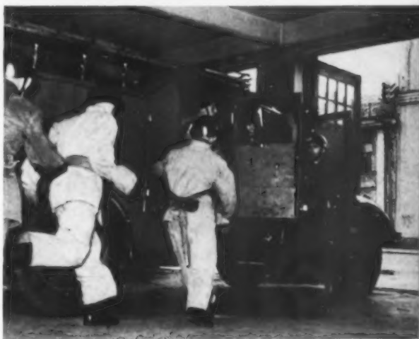
EQUIPMENT AND MEN ARE EVER READY FOR ACTION.
