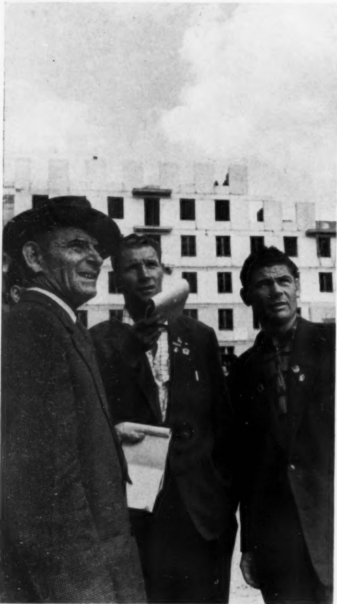
DIETHERLANDERS OF THE BUILDING TRADES INSPECT A MOSCOW HOUSING PROJECT.
