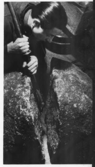
This discharger, designed by Lev Yutkin, splits a block of granite in a matter of a few seconds.
