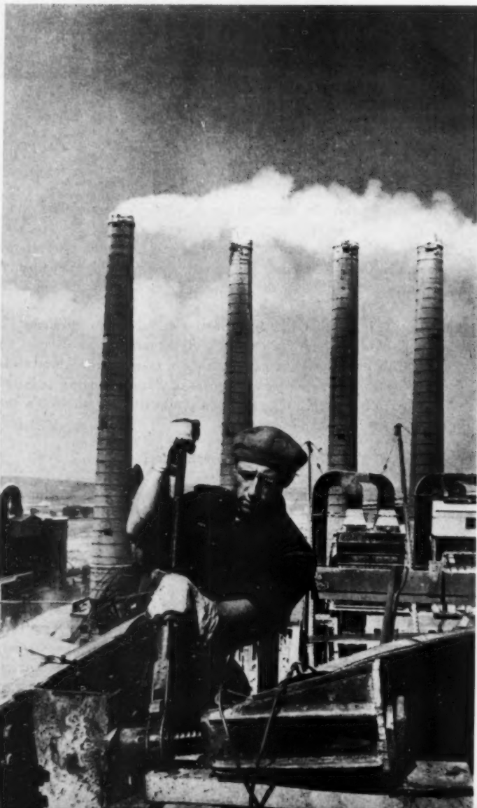
PLANNED CONSTRUCTION REQUIRES MANY NEW CEMENT PLANTS LIKE THIS ONE.
