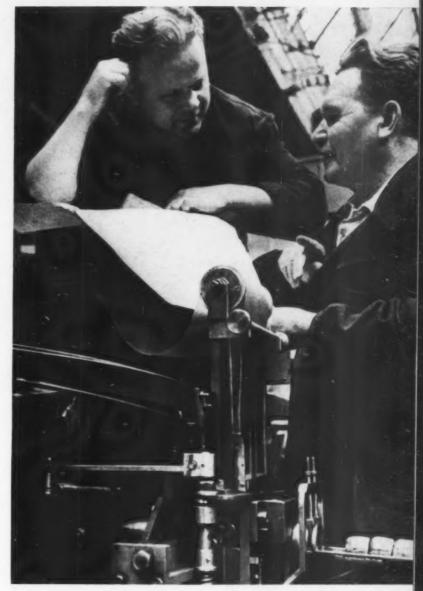
Alexei Viktorov and Pavel Gorokhov and two other mechanics designed an automic machine that greases and packs shaft bearings.
