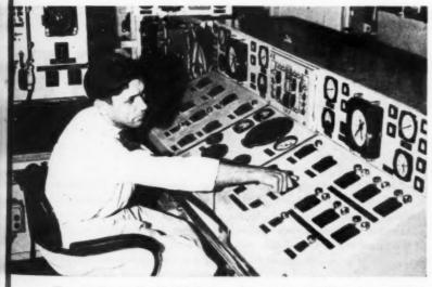
The atomic reactor installations, sealed and operated by remote control, are designed to protect the crew from exposure to dangerous radiation.
