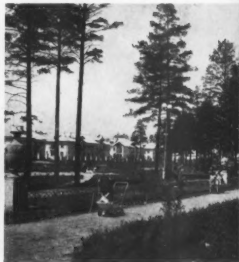
For builders of the Angarsk Hydroelectric Station—East Siberia
