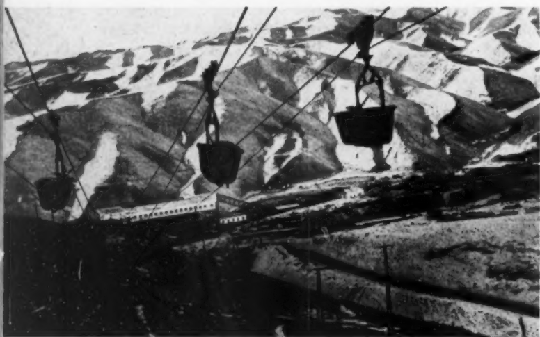
Cable-way buckets carrying zinc and lead ore for refining from the Altyn-Topkan mines, the republic's big nonferrous metallurgy center.
