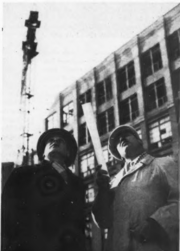
Deputy Malinkin checks on construction progress. He makes periodic reports on his legislative work to his constituents.
