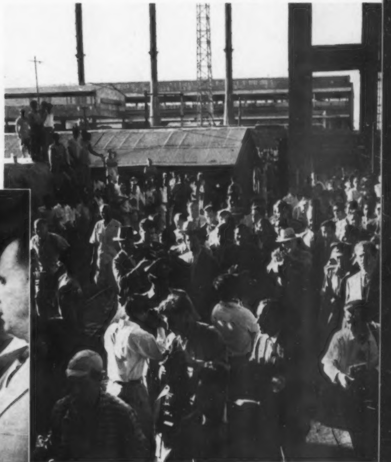
SOVIET-INDIAN COOPERATION BUILT THE GIANT BHILAI STEEL PLANT.
