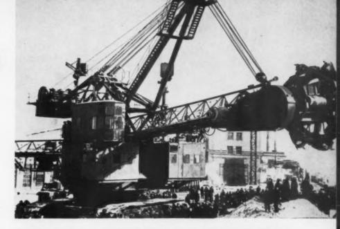
The plant makes this continuous-action rotary bucket excavator used for opencast coal and iron ore mining.
