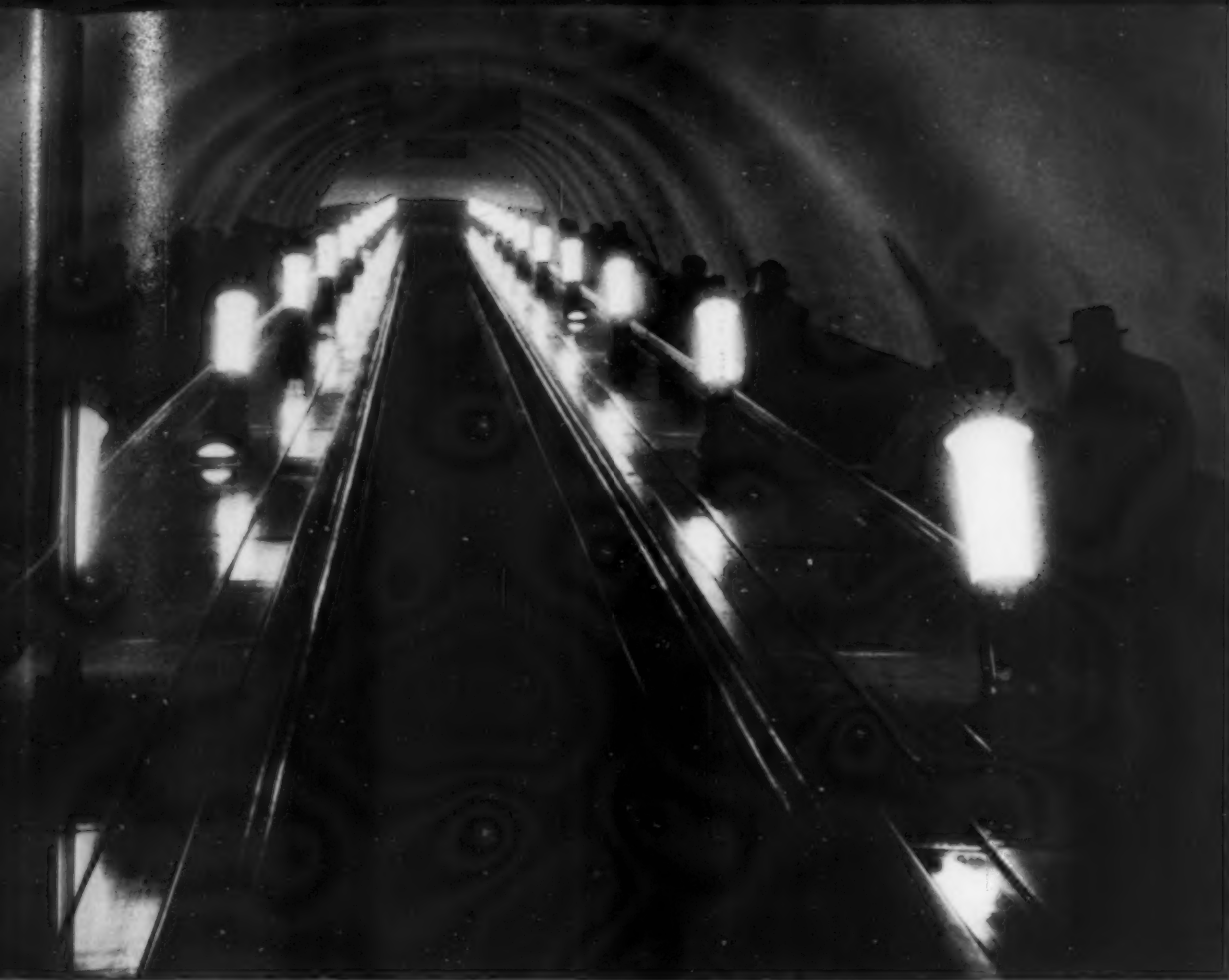
Most of the Metro lines are built quite deep, with escalators from street to station as long as 200 feet and more.
