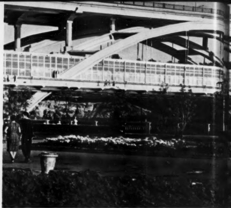
Lenin Hills Station is built on a bridge across the Moscow River with exits on both banks. The upper tier is used for auto traffic.
