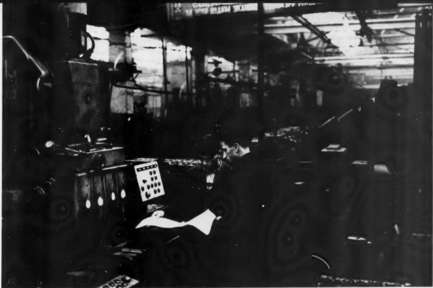
1. This transfer line to finish cylinder heads designed for the Minsk Tractor Plant does three times the work with fewer operators. Here electrician Alexander Mamai (right) and engineer Vladislav Maimusov check it's operation to see what improvements can be made. The new line eliminated the jobs of a number of men, who were all transferred to new jobs after retraining. 2. Victor Sheban is now working as a technician with a group of designers who are expanding the engine shop. 3. Vladislav Gudkovsky is in the chassis shop. The new jobs pay no less than the old ones did.
