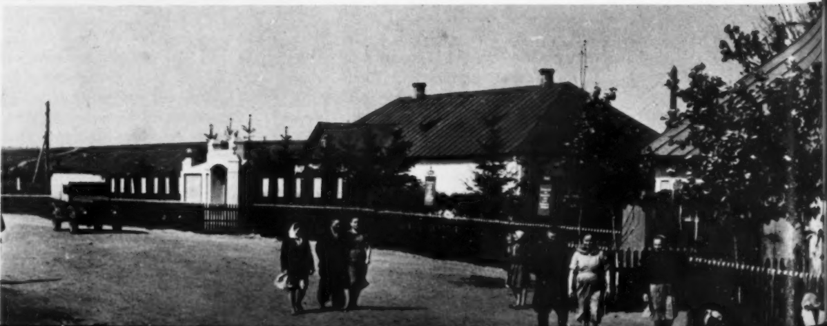
The farm has been doing a great deal of building since the merger. One of the new streets in this growing community.
