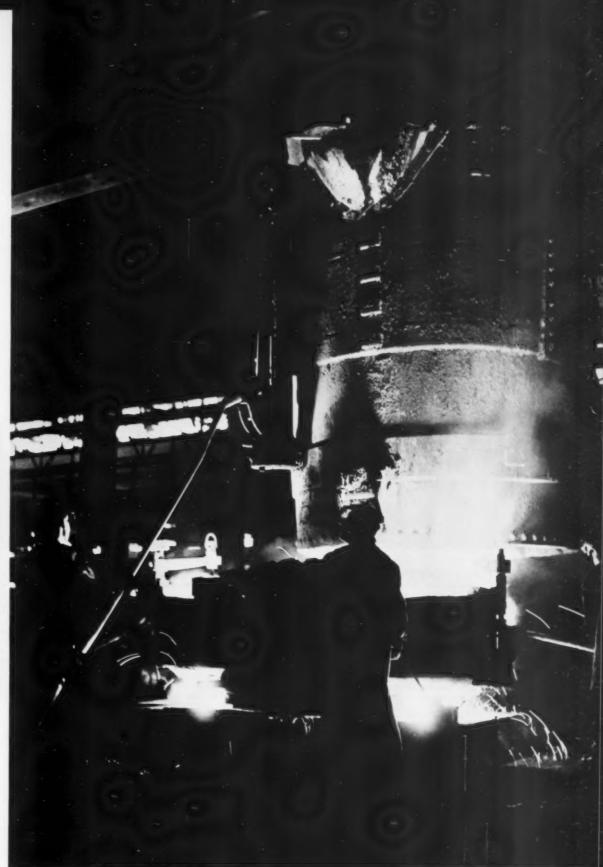
The continuous steel pouring installation at the Krasnoye Sormovo Mill has increased production and cut the work load.
