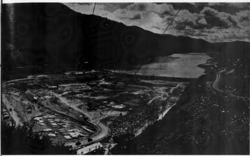
Site of the future Krasnoyarsk Hydroelectric Station on the Yenisei. The foundation pit has been built and is being prepared for the first concrete pour.
