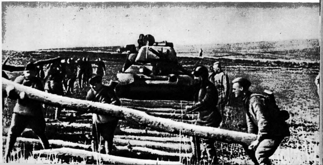
Sappers lay flooring for tanks, 1st Ukrainian Front, April 1944
