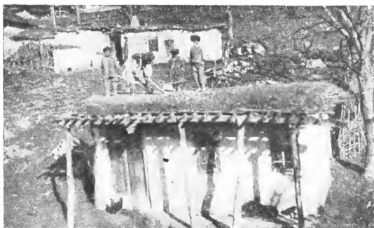
Grozny. A Chechen's hut in the "Old Oil-Fields"
