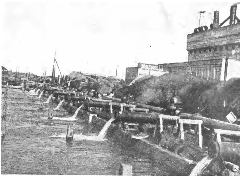
The Kuznetskstroy. Cooling basin of the Central Power Station
