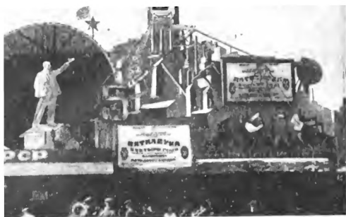
The drawing of the "Five-Year Plan in four years" loan in Ukraine. Decoration of the building where the drawing takes place
