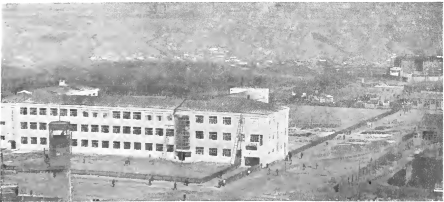
Stalingrad Tractor Plant. New building of the factory apprentice school
