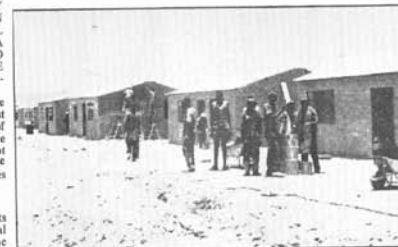
African building teams at work on houses in the new location.
