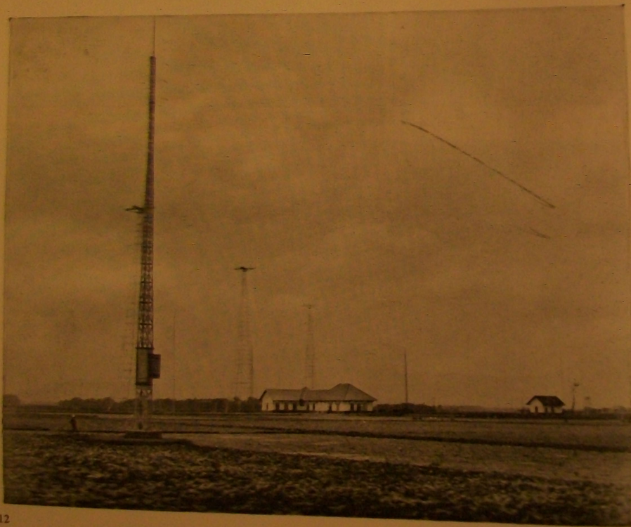
Broadcasting Station in Bandung
