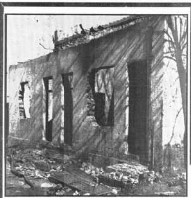
LEFT: This shell of a house was all that was left of the Resha's home in 134 Good Street, Sophiatown, after the Resettlement Board demolition team had done its work.
