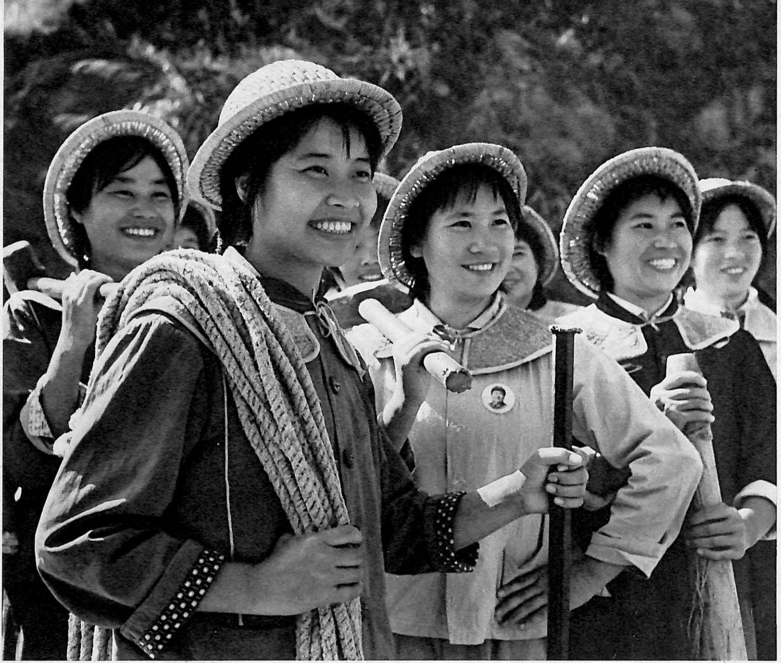
At the Construction Site.
