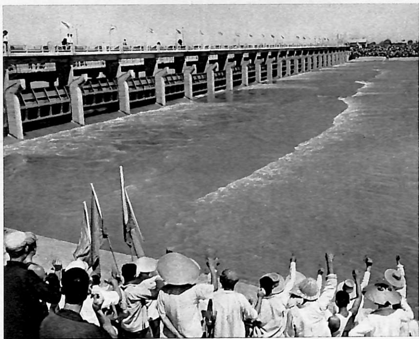
The Tsaolinchuang junction project on the Taching River near Tientsin. Harnessing the river has freed farmland on the banks from flood and waterlogging.
