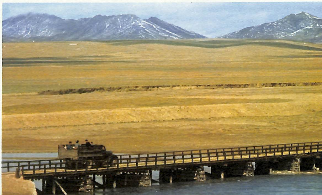
A bridge built by the Kyareng Lake commune, Matod County. This is the first bridge in the upper reaches of the Yellow River.
