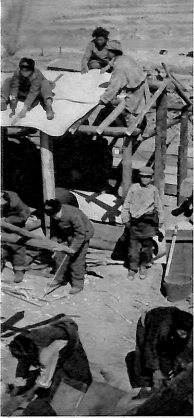
Armysmen and civilians put up wooden sheds for temporary shelters.
