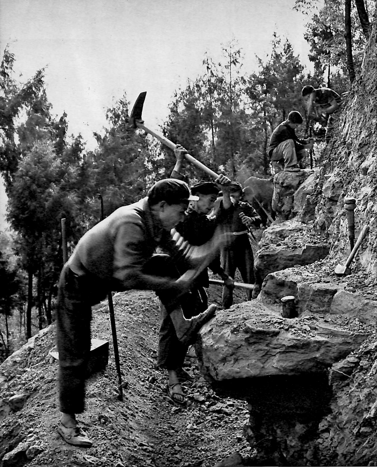
Building a canal through the mountains.
