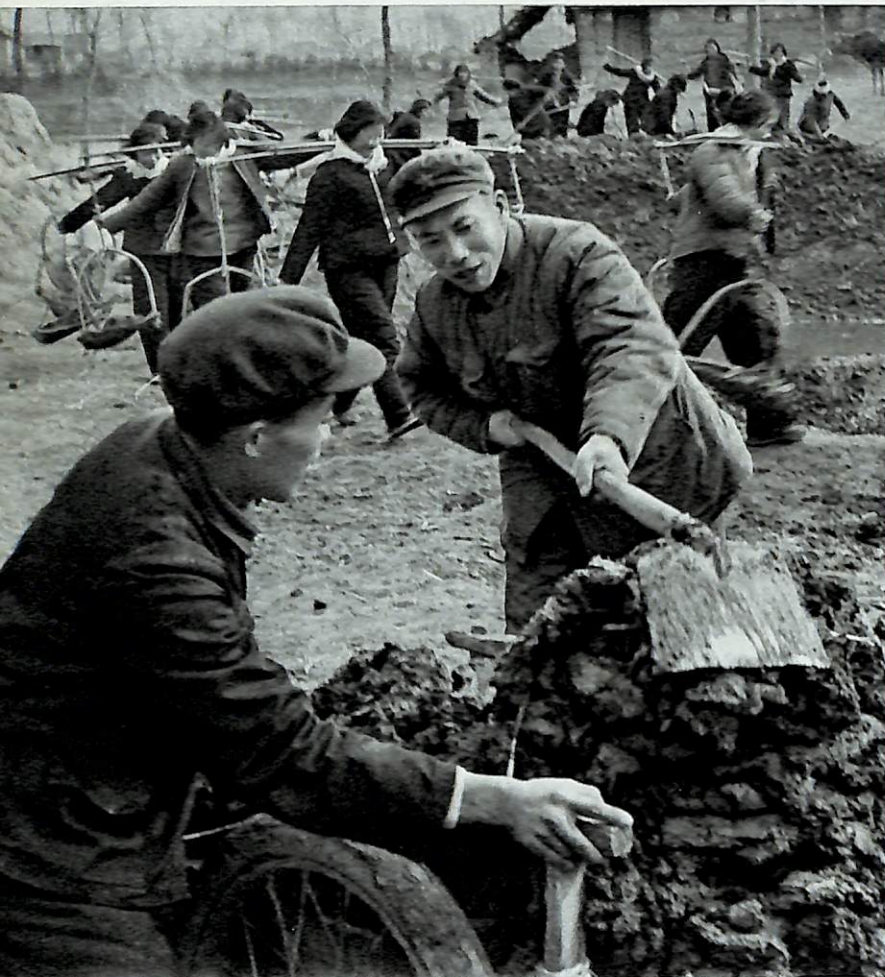
Doing farmwork with the commune members.
