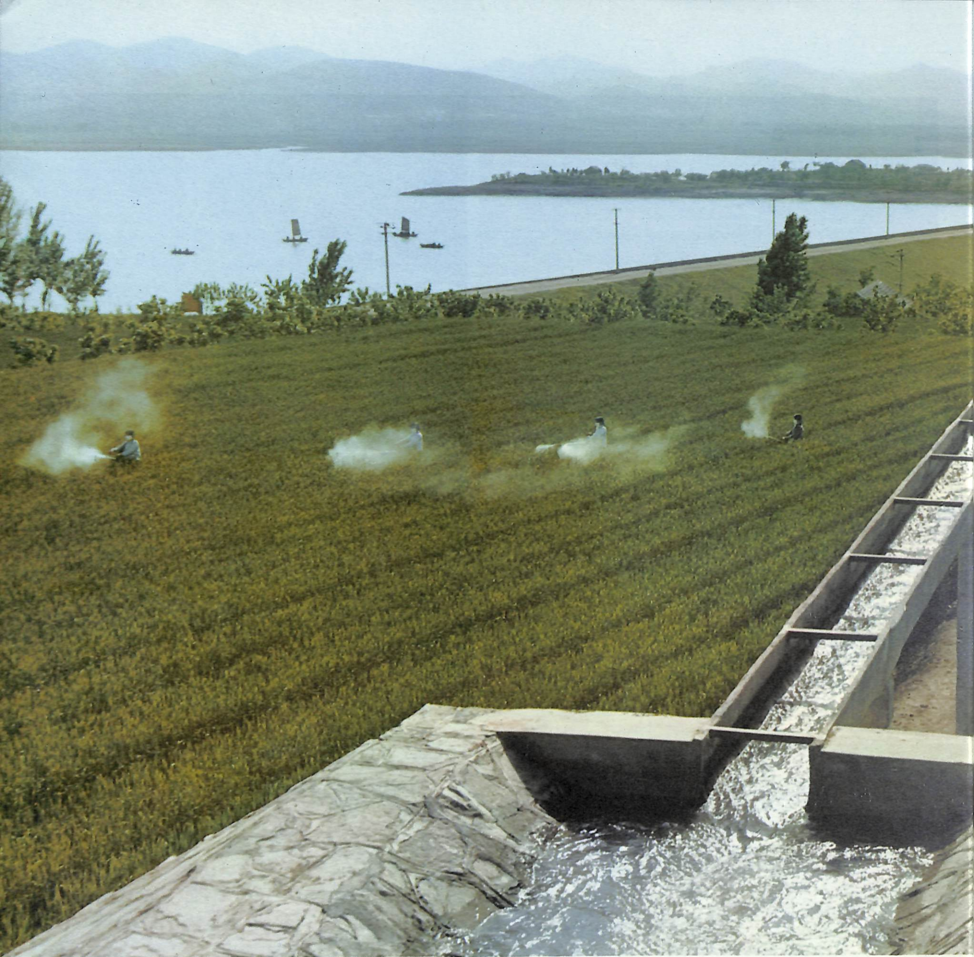
Part of the areas irrigated by the Yehyuan Reservoir, built in 1958.
