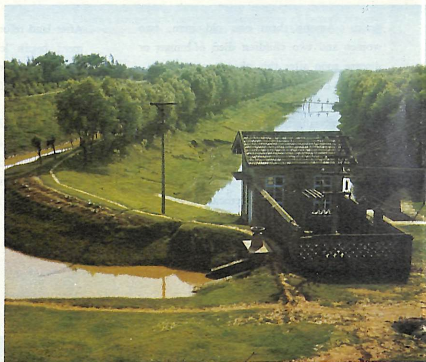
Electric power station for irrigation and drainage built during the Great Proletarian Cultural Revolution.
