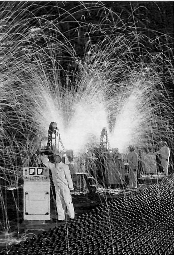
Welding anchor chains. By Li Sheng
