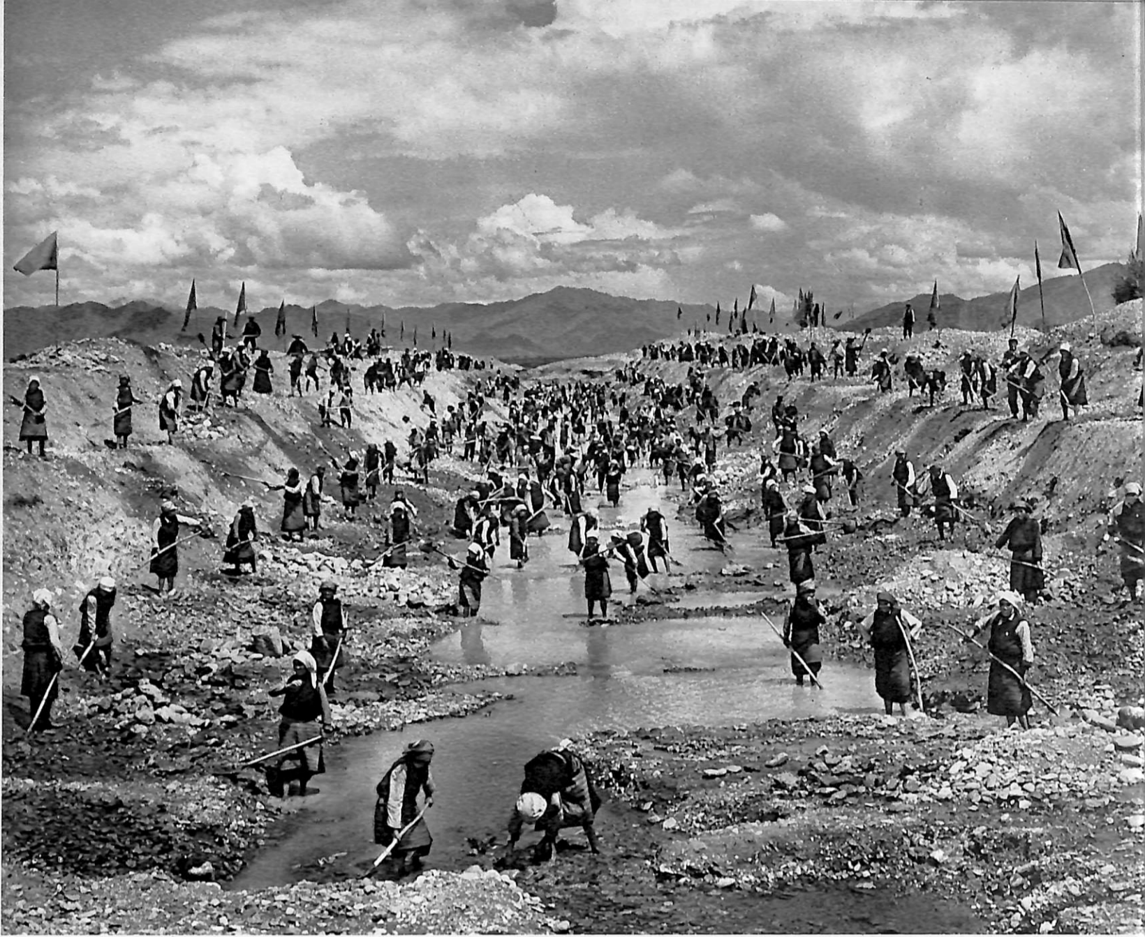
Working on a water conservancy project.
