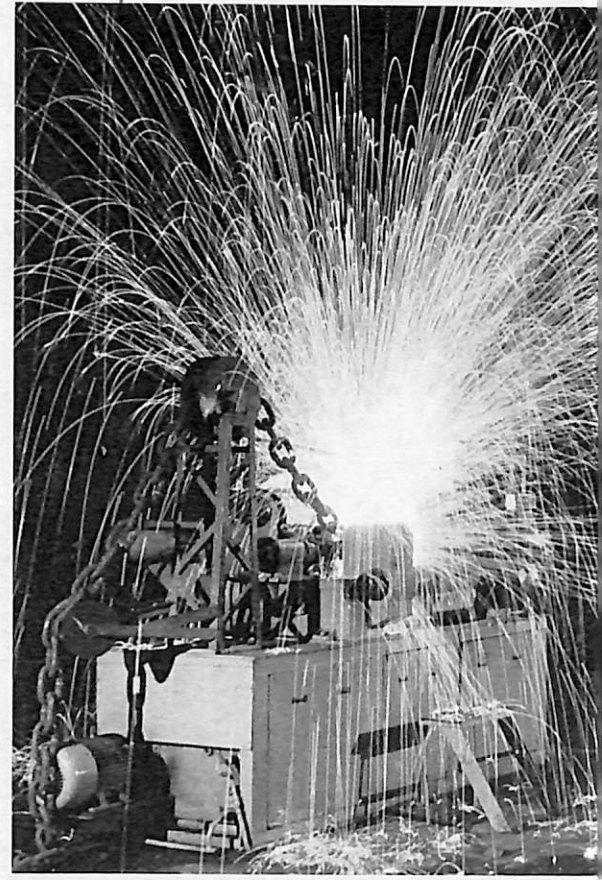
High-speed mechanical tunnelling. By Chang Chih-ming
