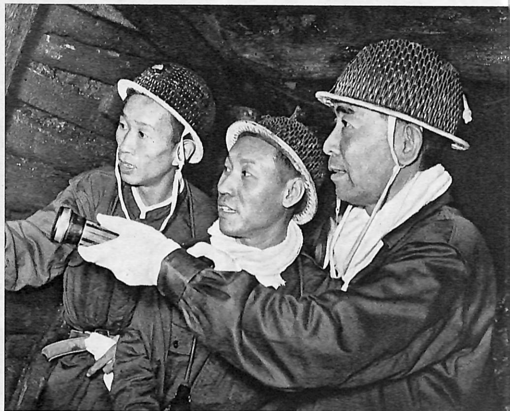
Premier Chou En-lai inspecting hydraulic coal drilling at the Tangchiachuang Mine of the Kailan Colliery, 1958.
