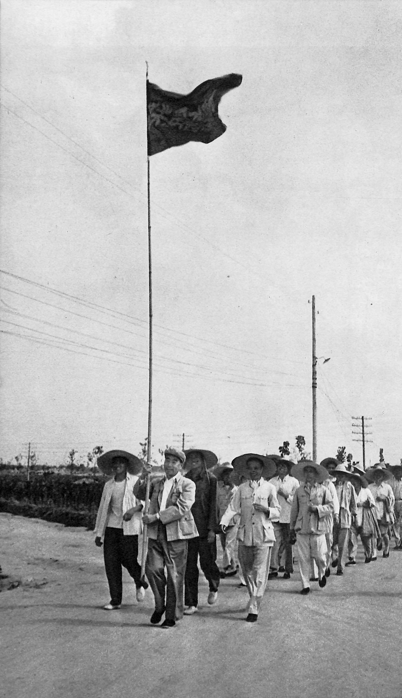
Holding high a red flag, Premier Chou En-lai led responsible comrades of the departments under the State Council to work at the Ming Tombs Reservoir construction site, June 1958.
