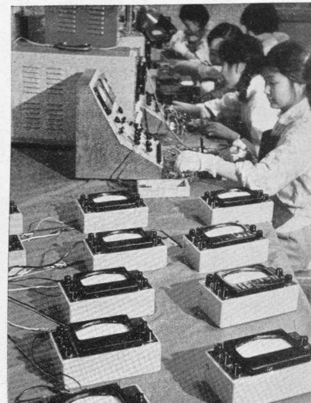
Testing the gauges at the Chungyuan Electric Plant in Shanghai. Hsia Tao-ling
