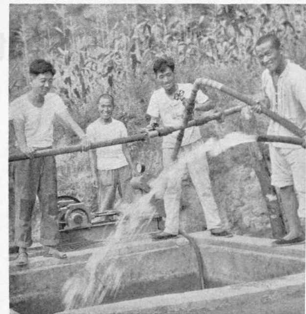
Pleasant interlude while helping commune members install a water pump.
