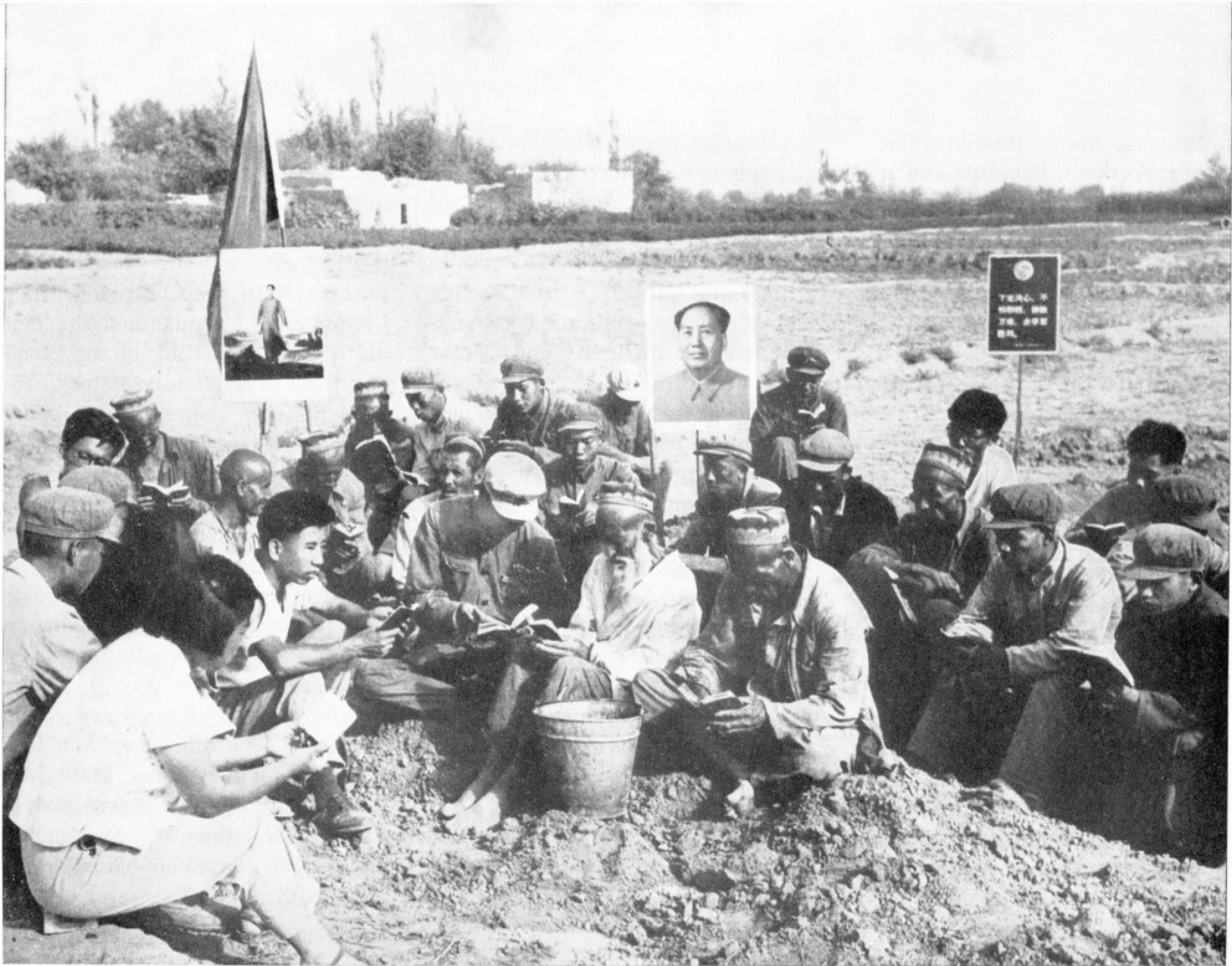
Members of the observation team, P.L.A. fighters and the local poor and lower-middle peasants study Chairman Mao's works during a break in installation work.
