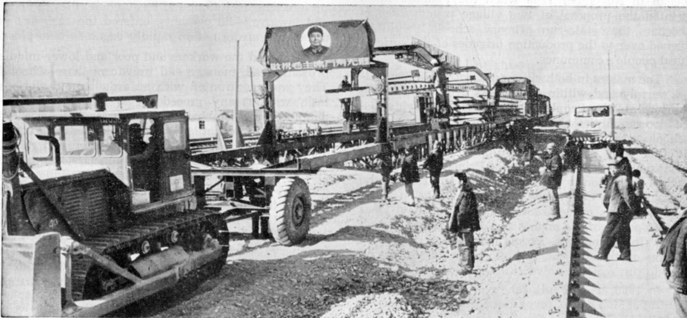
A new rail and tie laying machine designed and made by First Railway Engineering Bureau workers.
