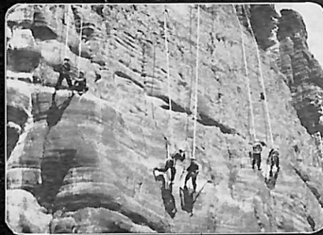
The canal will cross this cliff.
