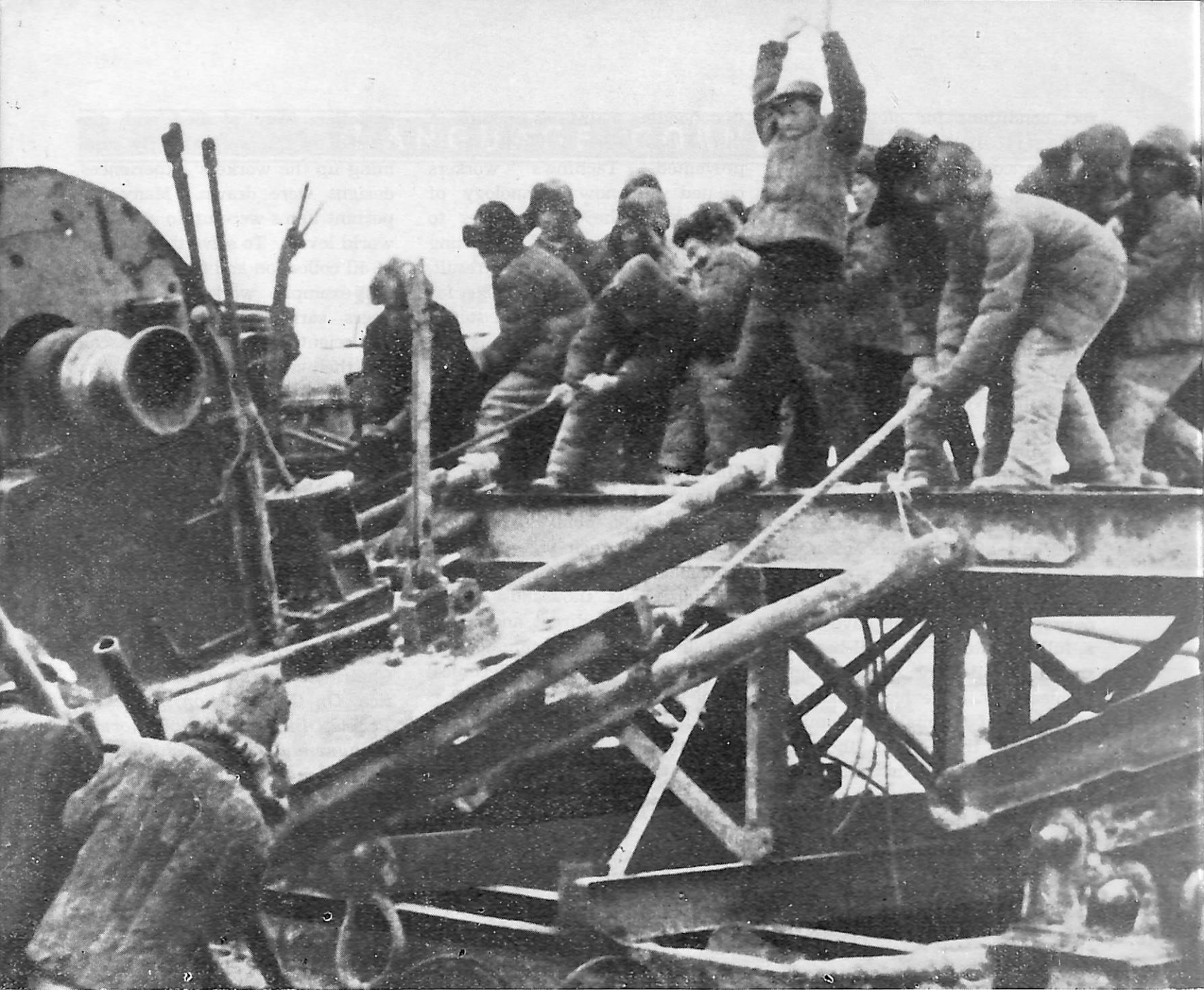
When cranes had not arrived, Drill Team No. 1205 led by Wang Chin-hsi moved drilling equipment with shoulders and crowbars.
