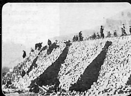
Making lime without a kiln.
