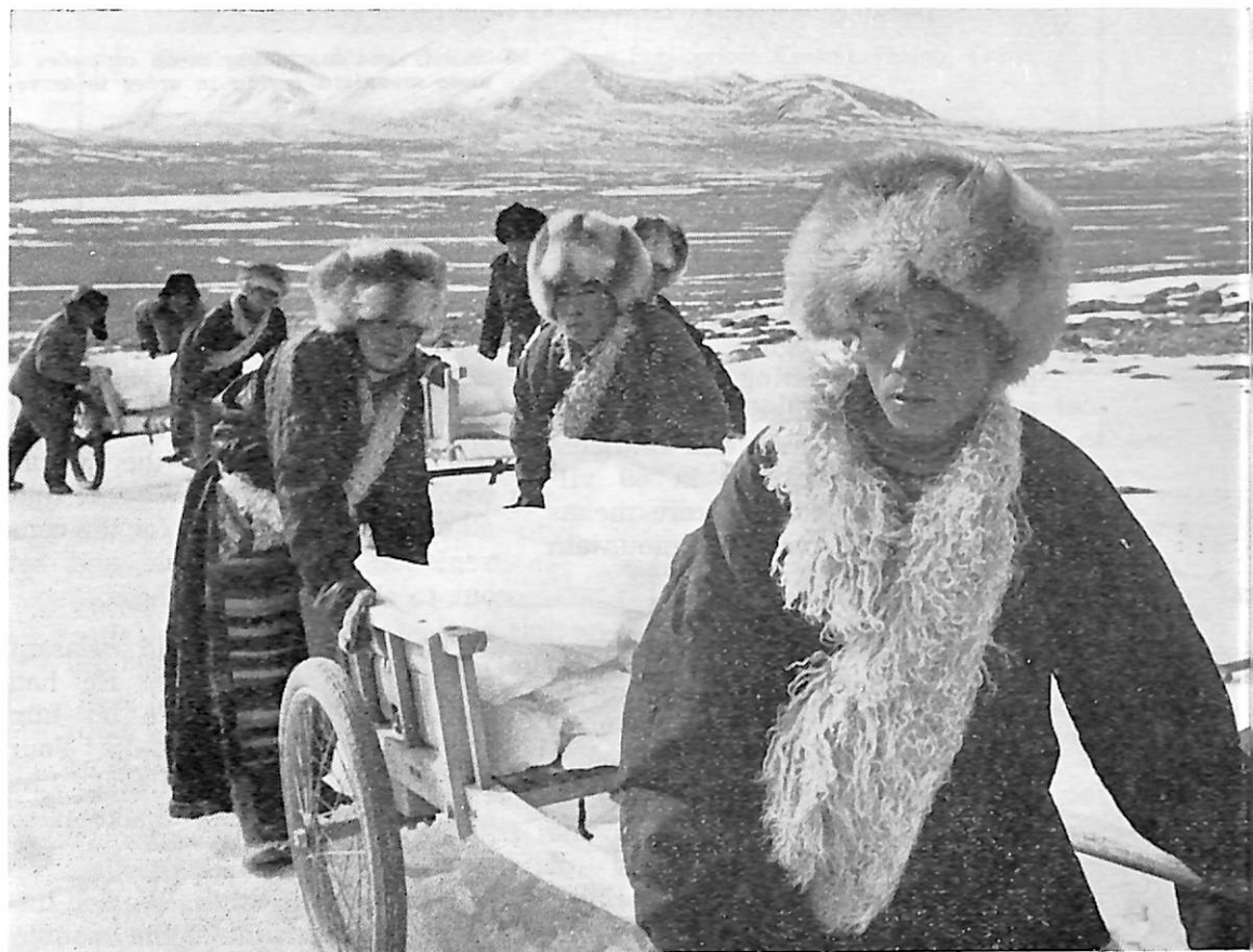
Clearing ice from the highway.
