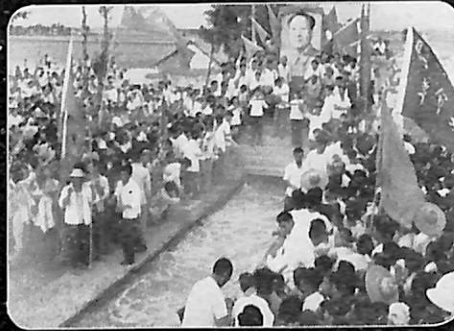
The opening of a trunk tunnel.
