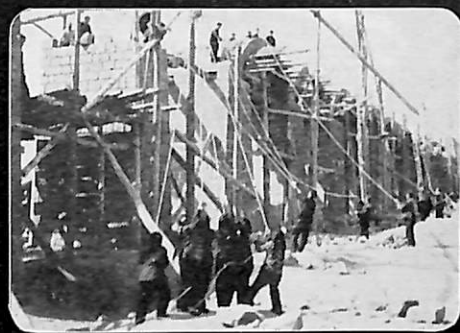
Lifting stones with an improvised derrick.
