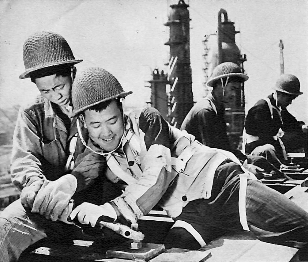
Installing refinery equipment.
