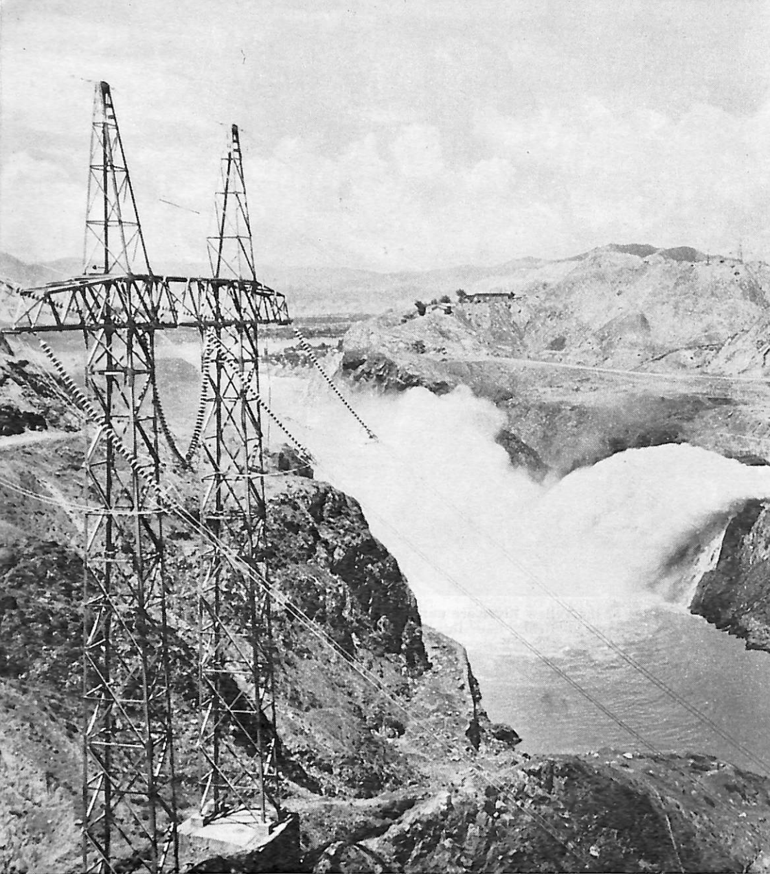
A large key water conservation project now completed on the Yellow River produces electricity.
