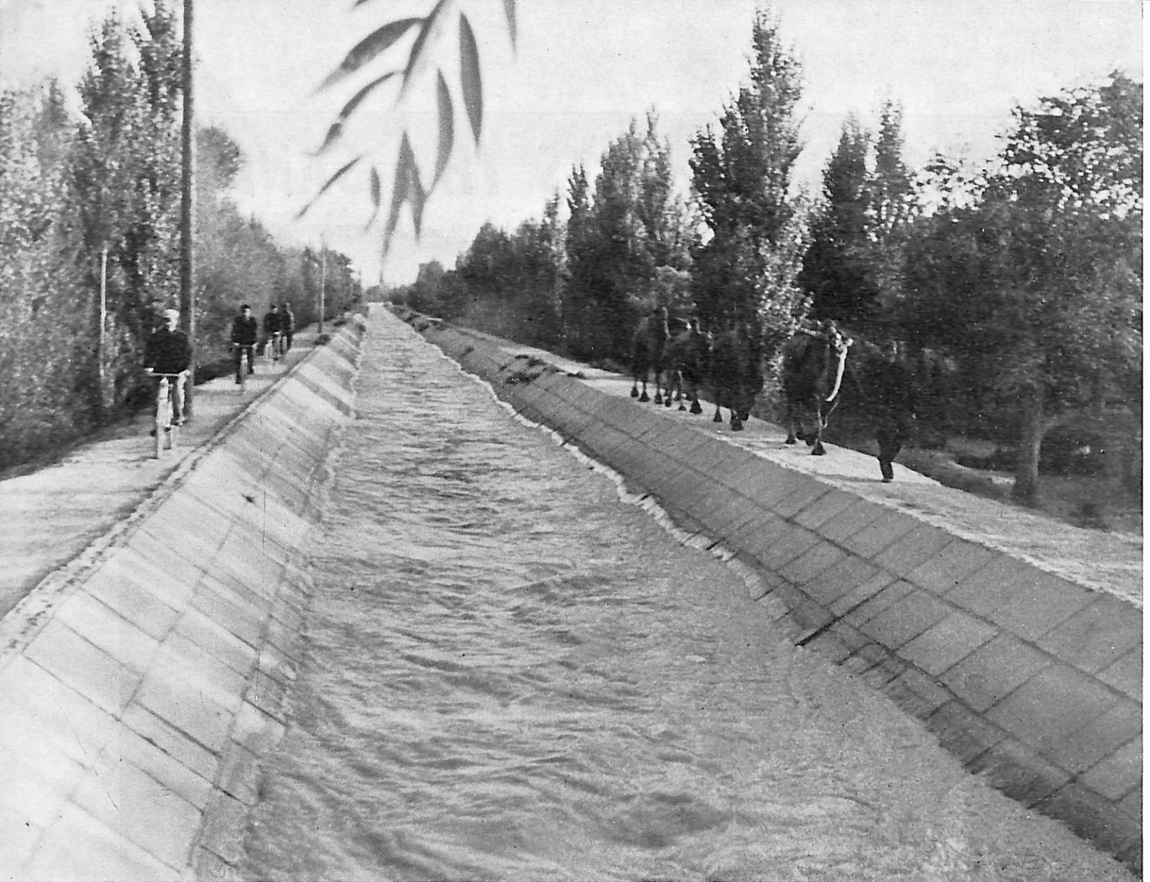
The new canal through the desert area carries water from the Tang River to fields all over the county.
