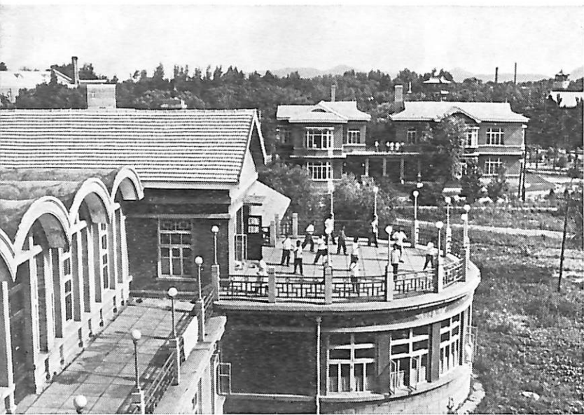
A section of one of the new buildings at the sanatorium.
