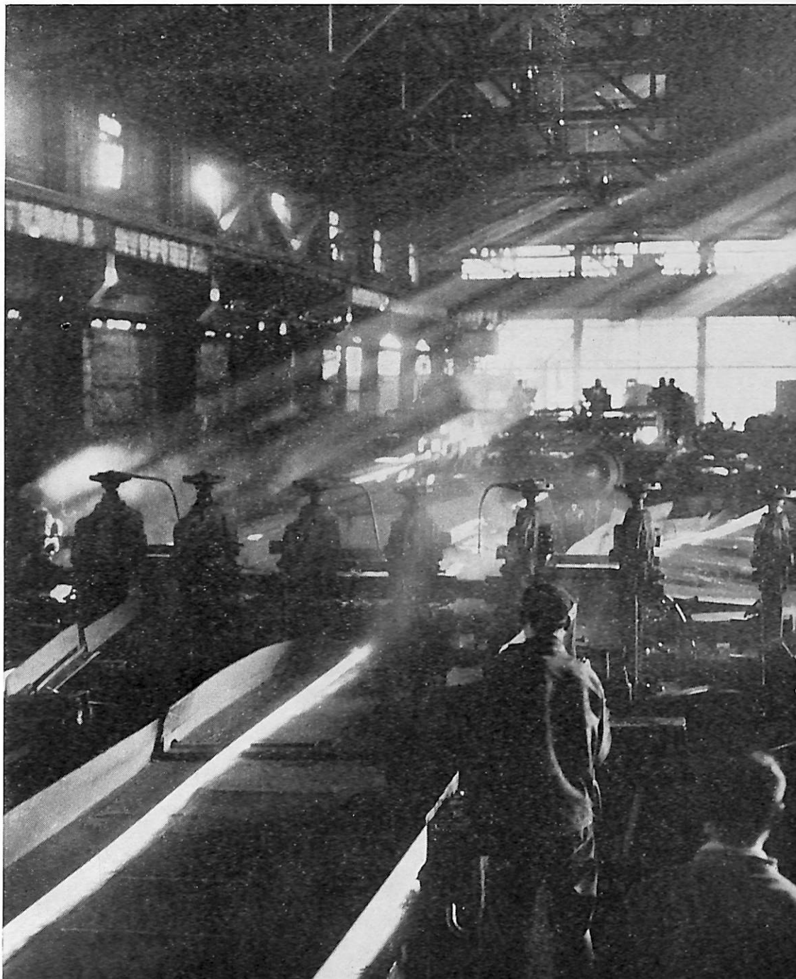
Inside the No. 2 Steel Rolling Mill.
