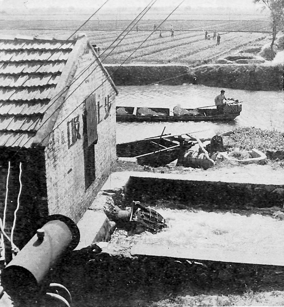
One of Chienhu county's pumping stations.
