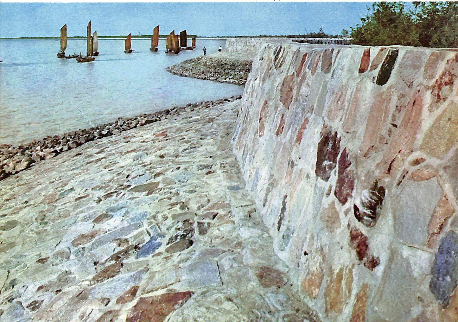
The stone dyke on the east bank of Kaoyu Lake.
