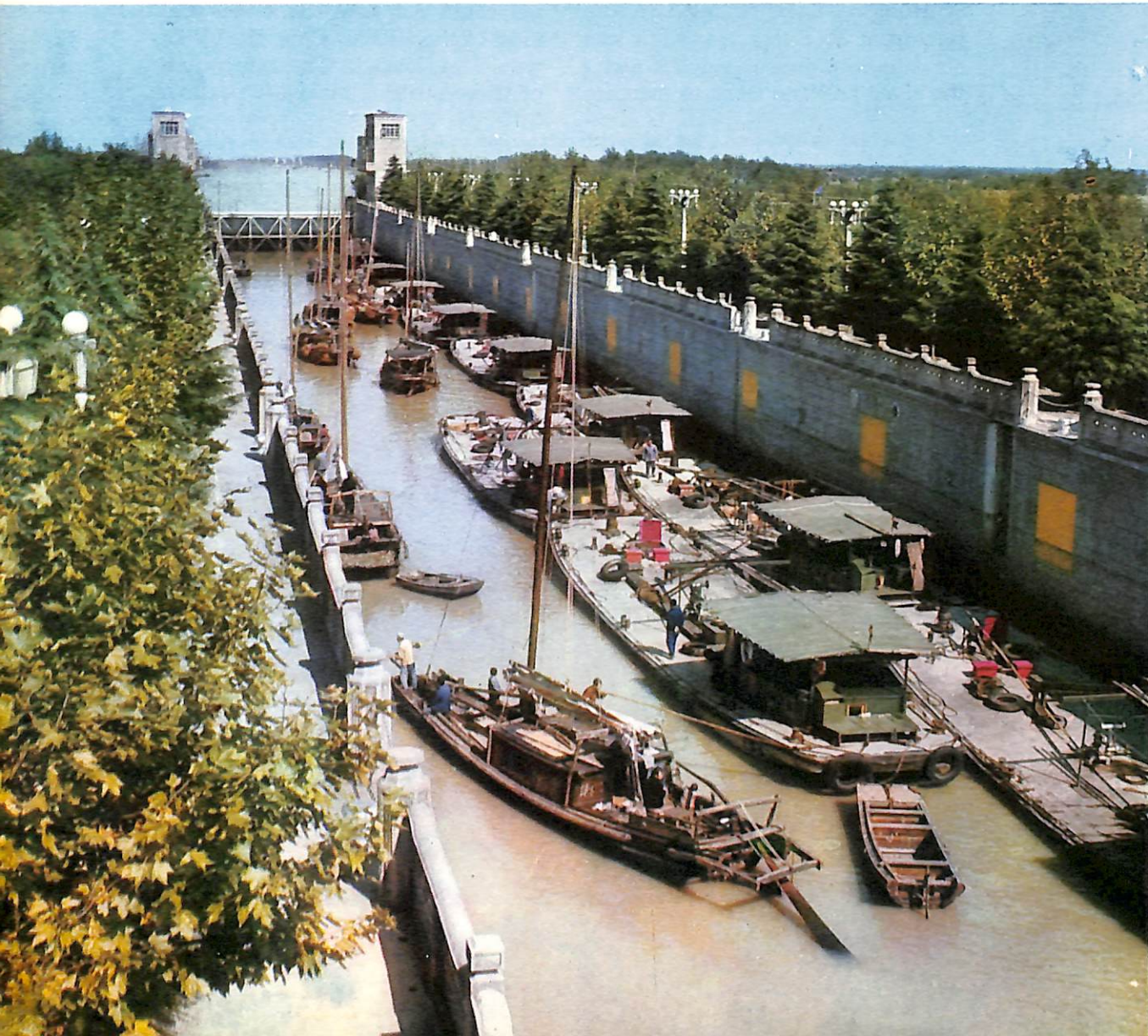
The Shihehiao boat lock as the Grand Canal enters the Yangtze also serves to regulate the level of the canal.
