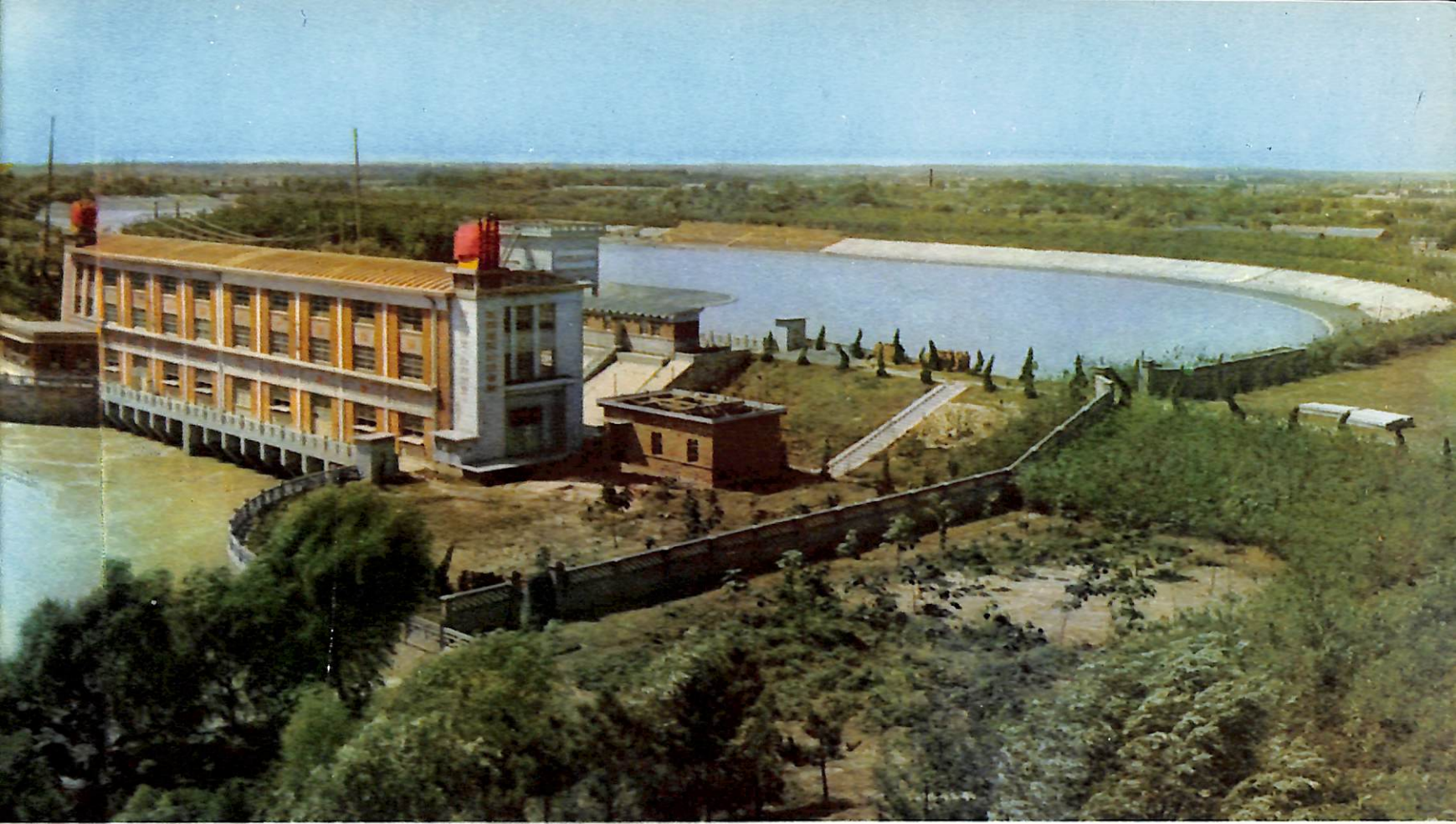
The pumping stations in Chiangtu.
