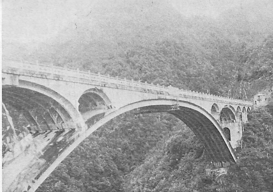
Open-spandrel bridge over a mountain valley.
