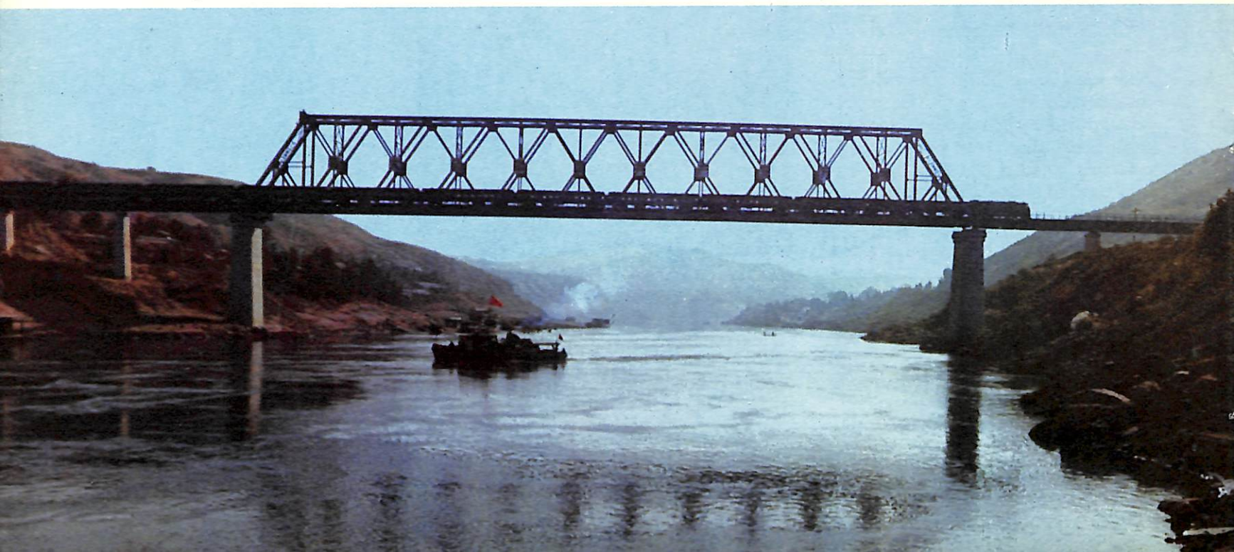
Steel bridge over the Chinsha River.
