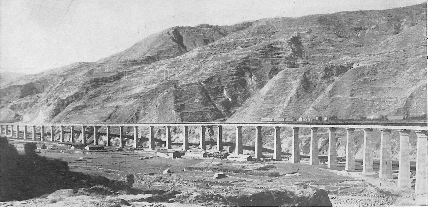
The Talienching Bridge, longest overpass on the Chengtu-Kunming line.
