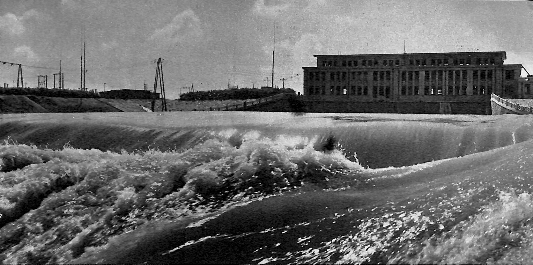
No. 1 pumping station of the Chiangtu water-control project on lower Yangtze.
