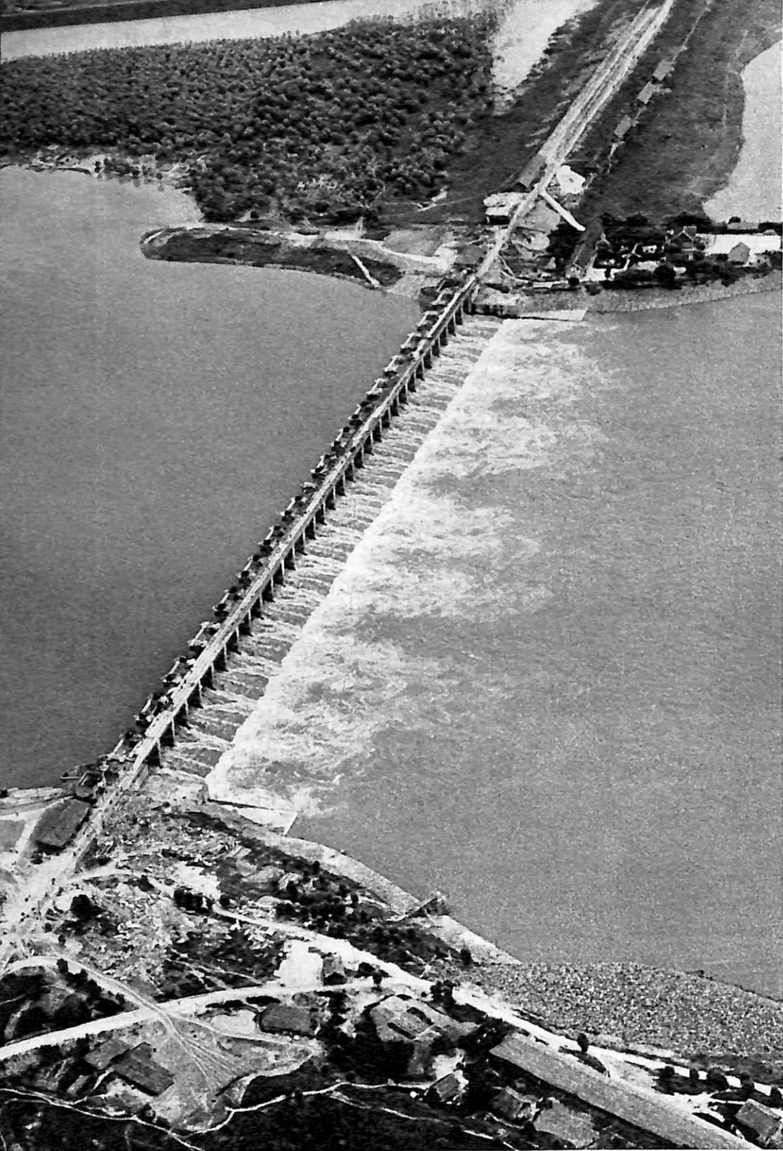
The Huangshantou distribution gate of the Ching River flood diversion project.
