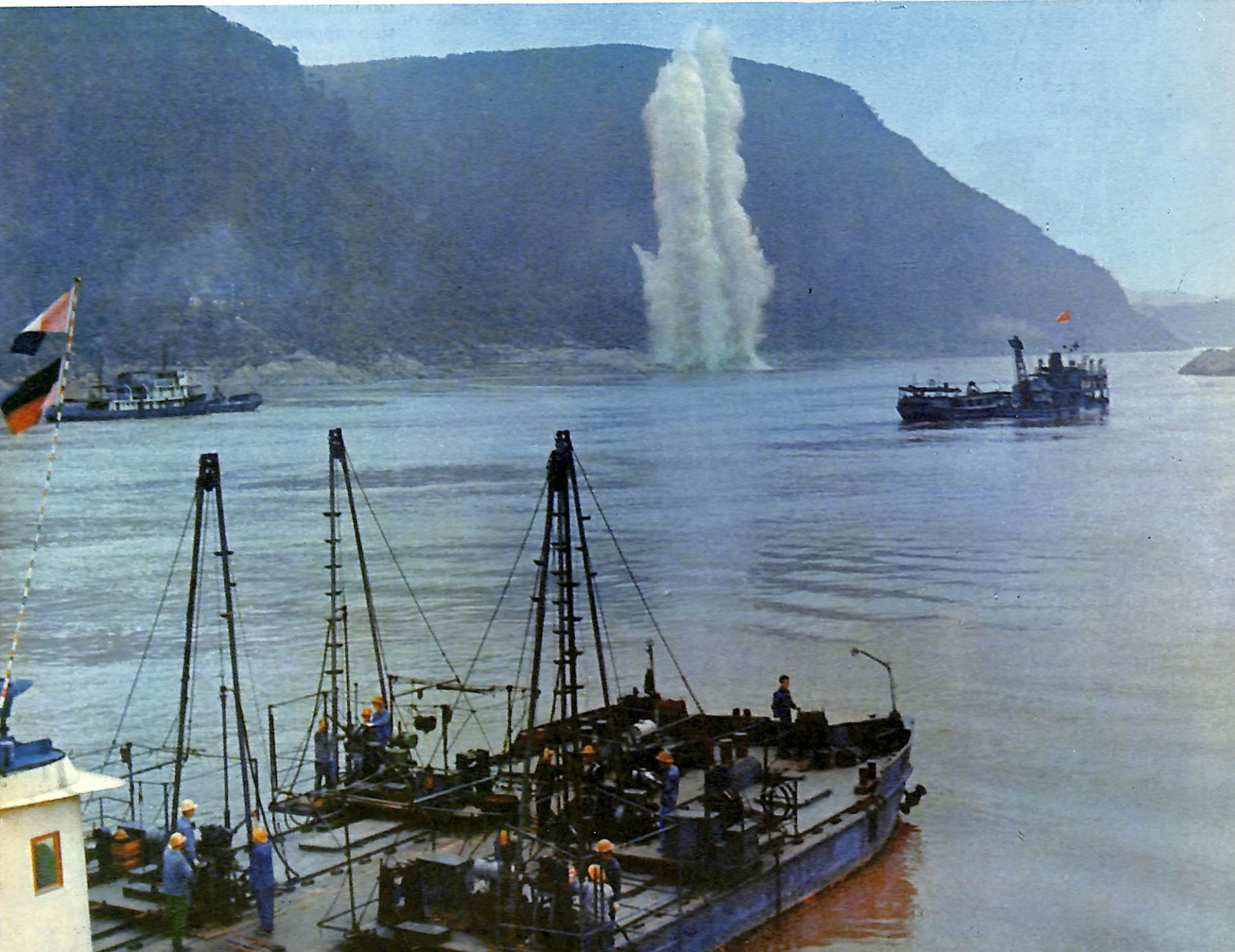
Blasting away a dangerous sandbar at the mouth of a gorge.
