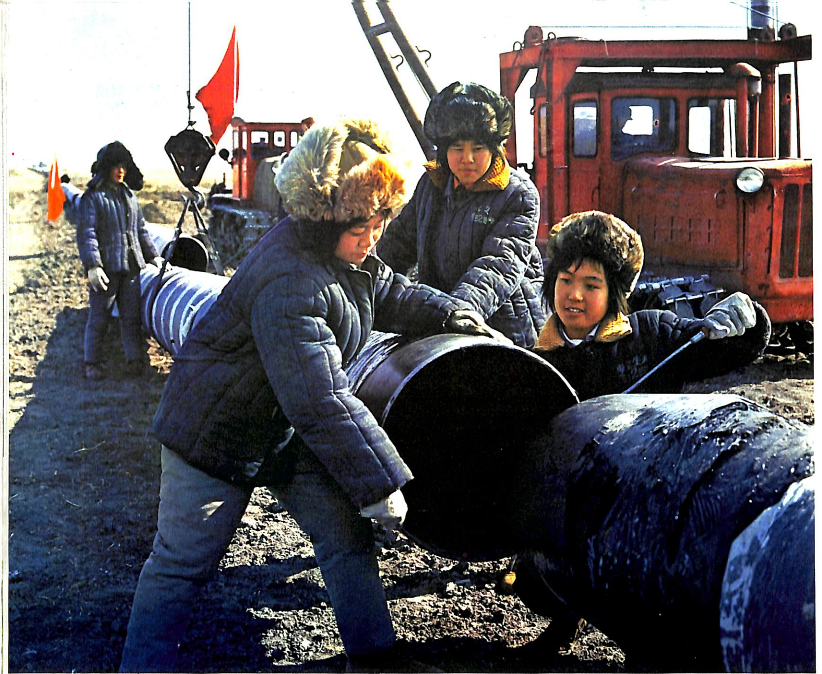
A team of women fitters laying a new pipeline.
