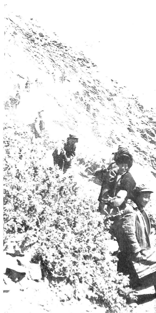
An 8.8-kilometer canal being built at 4,400 meters above sea level in Chhugo commune.
