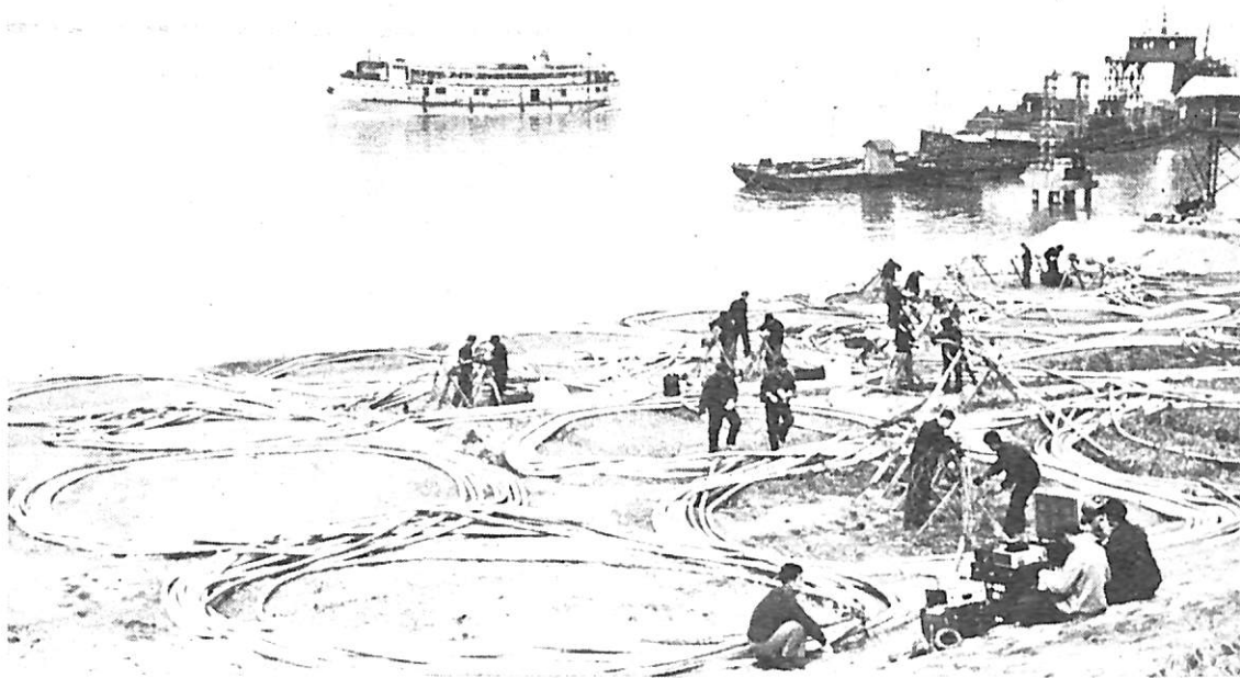
Testing coaxial cable before laying it across a river.
