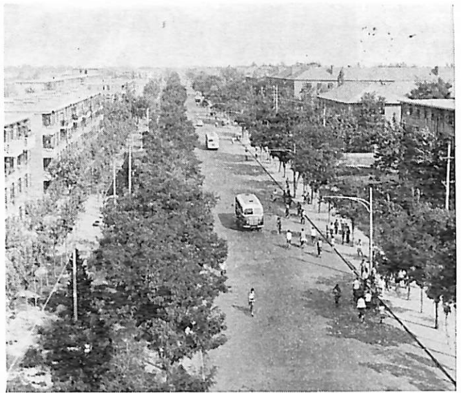
New workers' residential area.
