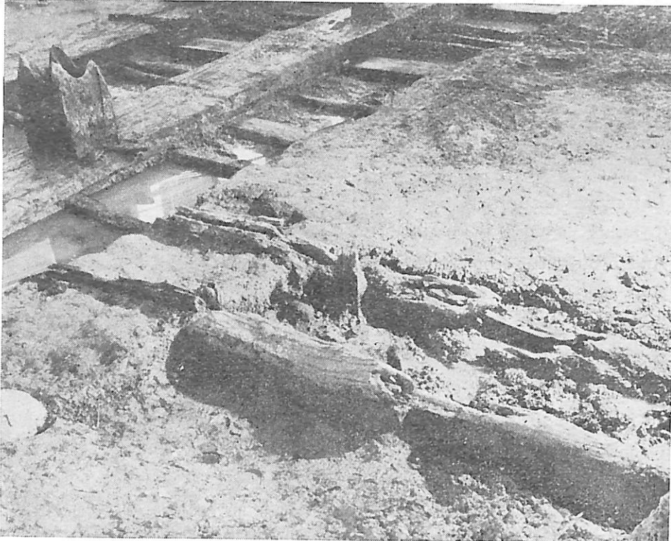
Device for bending timbers under heat.
