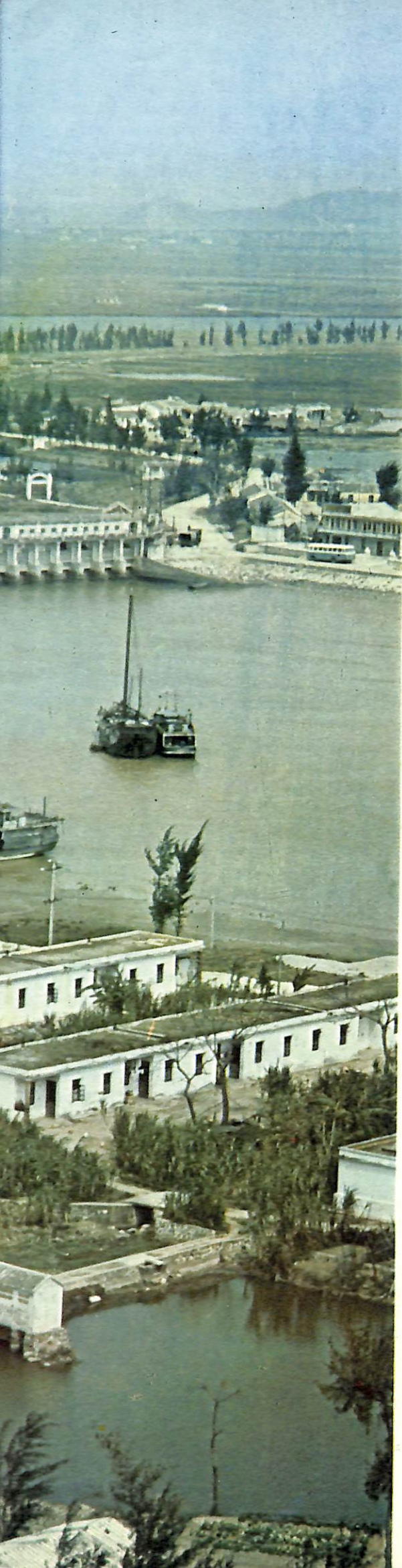
The 48-gate Fenghuochiao sluice.
