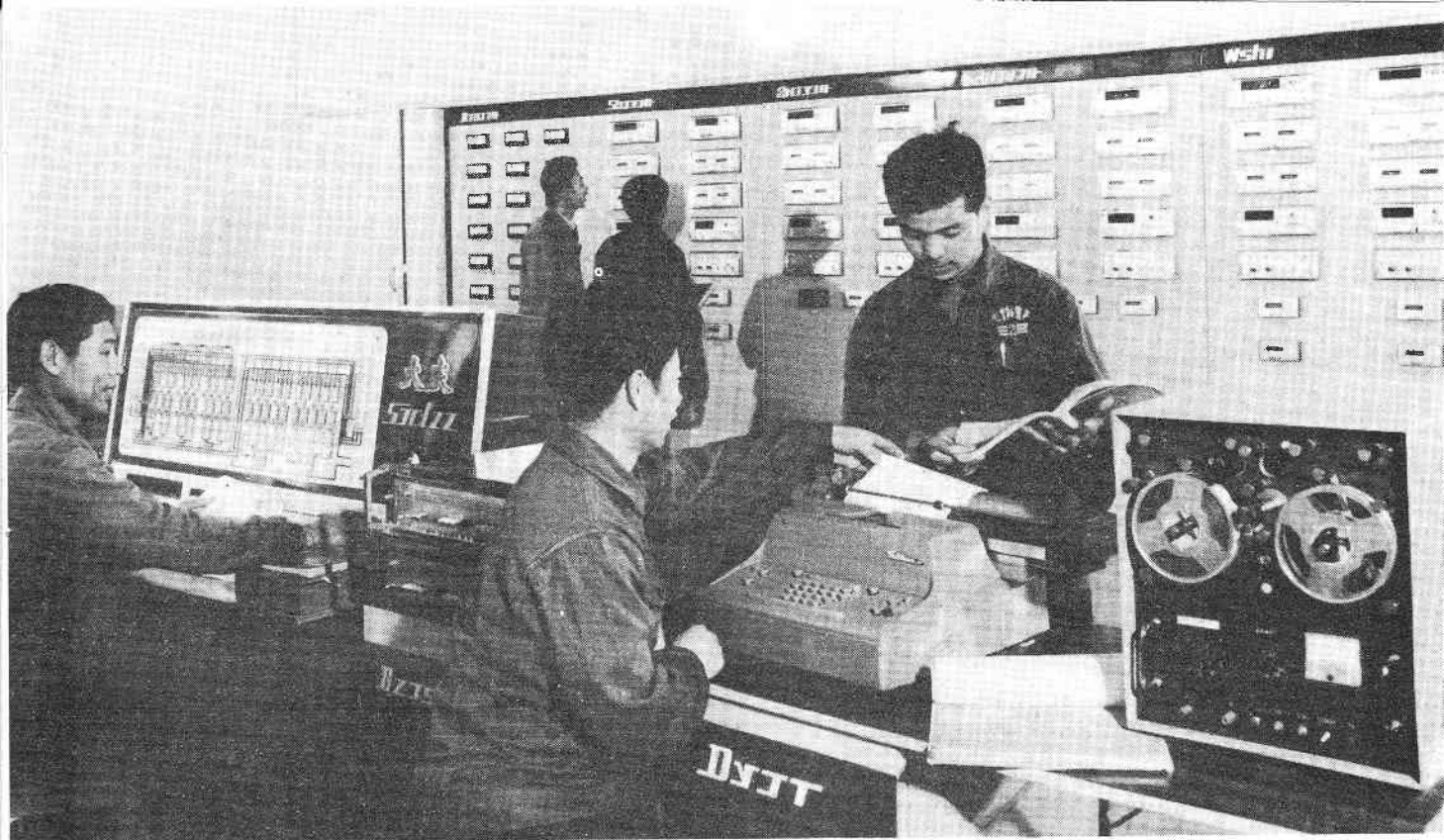
This control room in the main collection station tracks all oil flowing out of Daqing to other places.
