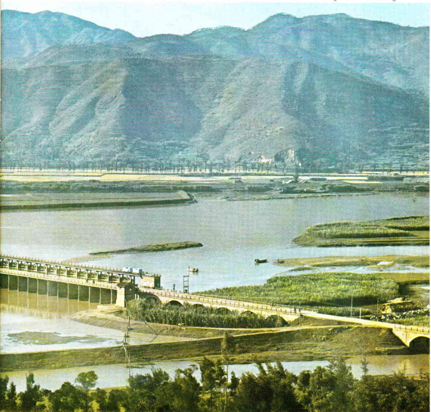
Jiulong River distribution gate.
